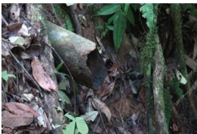
Photo: Gooseneck pipe forestuary drainage. Aguarico 4 wellzone. (12/09/2014)
